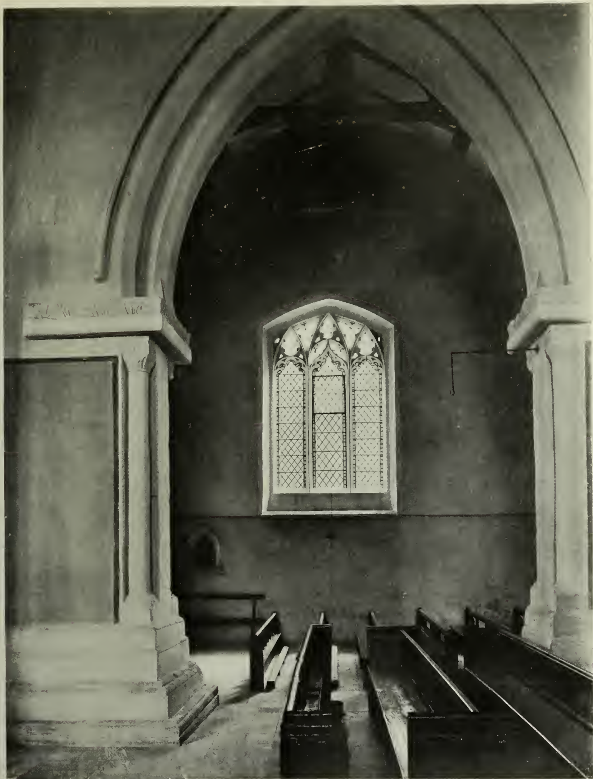
HADSTOCK : PARISH CHURCH OF ST. BOTOLPH. Archway to S. Transept; Responds, 11th-century; Arch, 13th-century.
